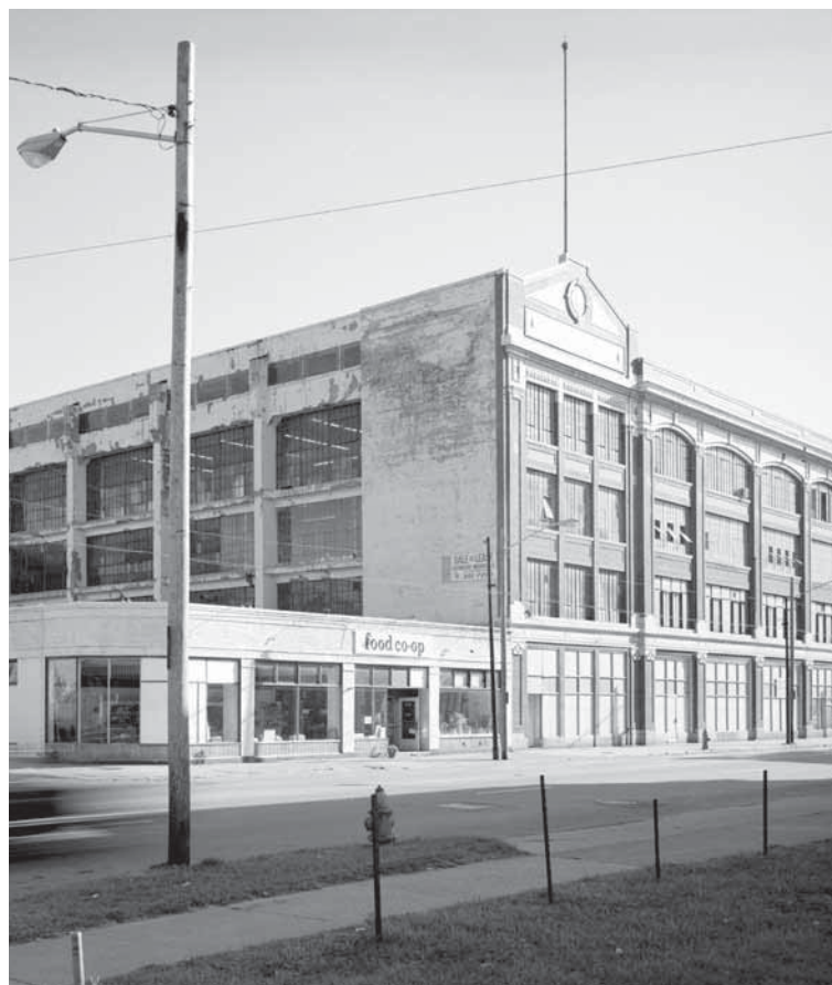
Cleveland Institute of Art (CIA) McCullough Center, Cleveland, Ohio: The Cleveland Institute of Art received a 2011 Preservation Award from the Cleveland Restoration Society and AIA Cleveland commending the renovation of the 96-year-old Joseph McCullough Center for the Visual Arts on Euclid Avenue. “We are delighted to receive this recognition from the Cleveland Restoration Society and AIA Cleveland,” said CIA President Grafton J. Nunes.
